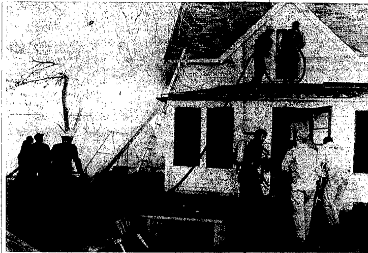
FIRE RAVAGED the Jack Hurlbut home at 527 E. 7th last Wednesday while the family was out of town. The fire apparently broke out in the living room and then moved up the wall to the upstairs. Firemen were hampered in their early efforts by heavy smoke and heat, as the house had been tightly closed. Very little of the family goods was saved as smoke and heat damage was extensive.
